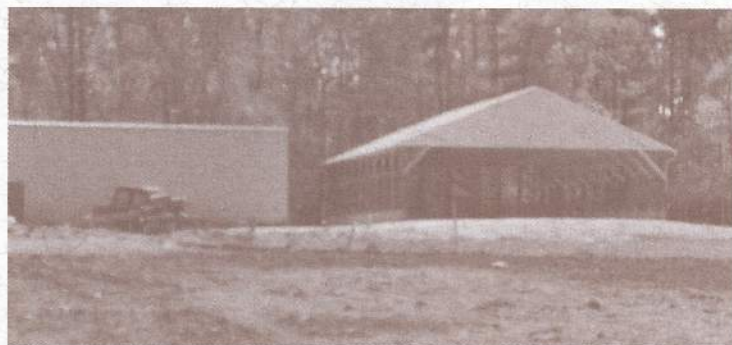
Recently Completed Manure Storage Facility
