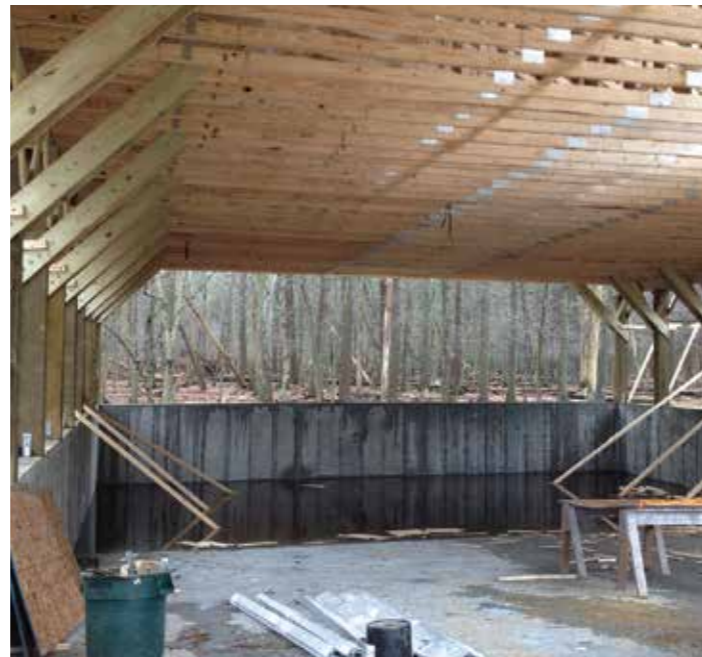
The Farm's Manure Storage Facility Nearing Completion
